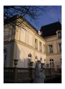
Rendering old building with lime mortars has been done traditionally to help keep the rain out, as part of local building practice to protect softer building materials below and for aesthetic reasons.
